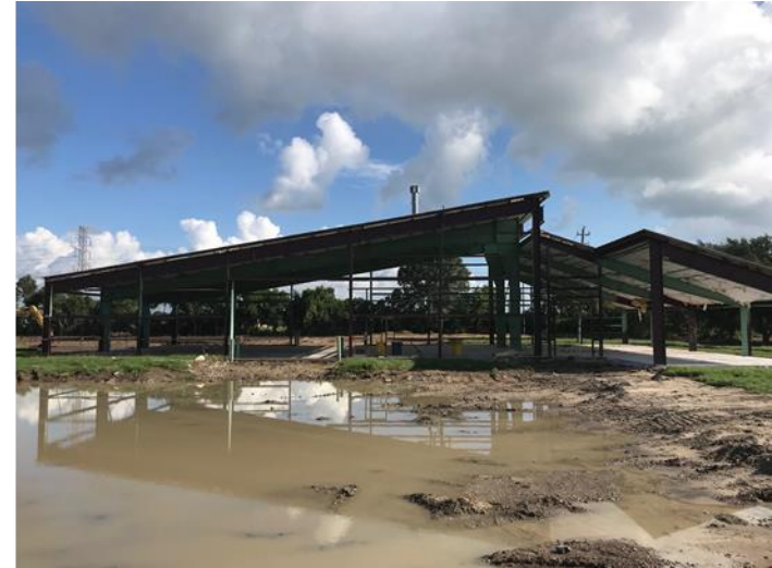
Automotive/Diesel Lab Renovations
