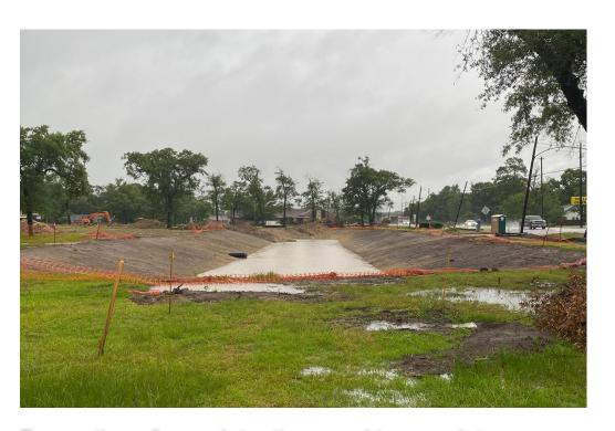
Excavation of new detention pond is complete
