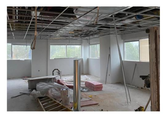
Metal framing & gypsum install is complete at the second floor, ceiling grid installation is underway
