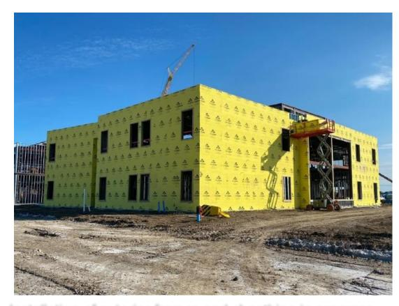
Installation of exterior frames and sheathing in progress
