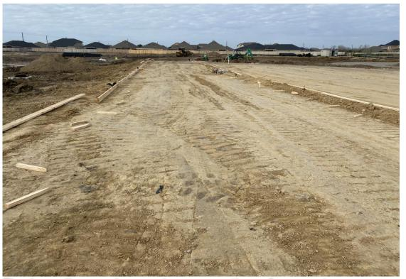
Final grading underway in preparation of concrete pour at parking lot
