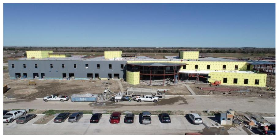
Installation of sheathing and waterproofing progresses
