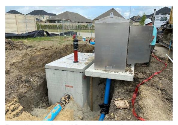
Domestic water line and fire line vault and meter box
