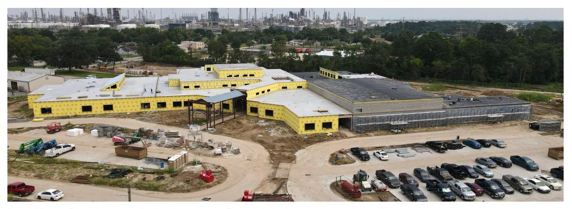
Aerial View – Sheathing installed and waterproofing underway
