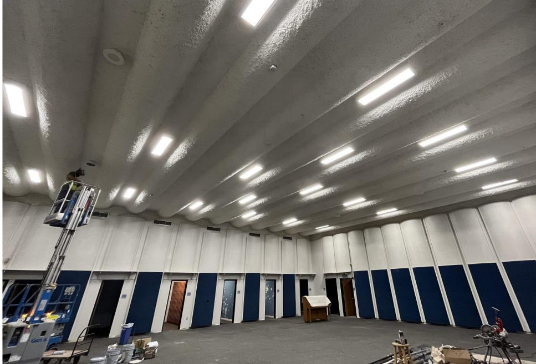
Sprinkler heads and speaker installation underway at the Band Hall
