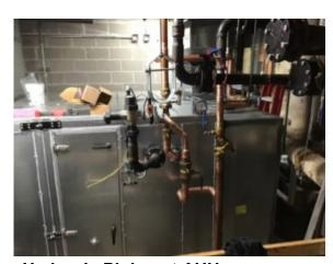
**Hydronic Piping at AHU**
