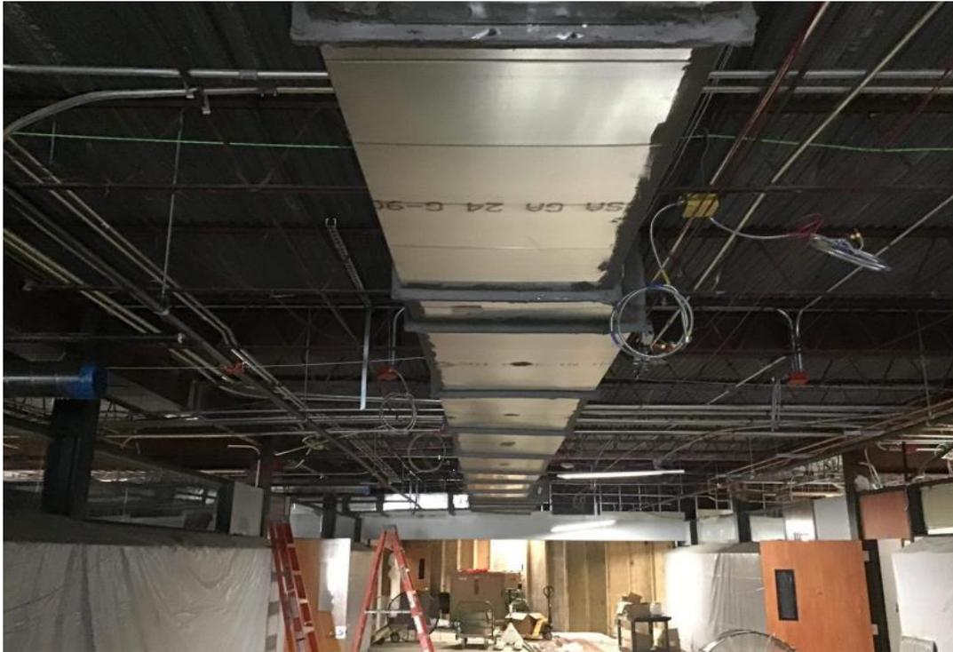
Medium pressure ductwork installation in Bio/Chem lab
