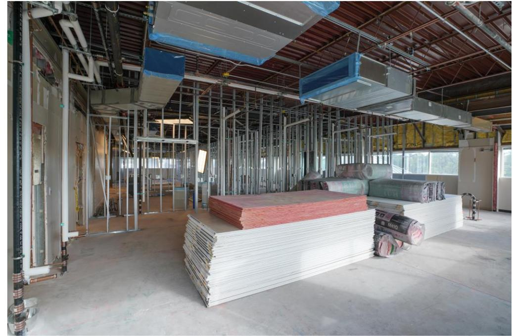
Metal framing is complete and is awaiting gypsum board installation on second floor
