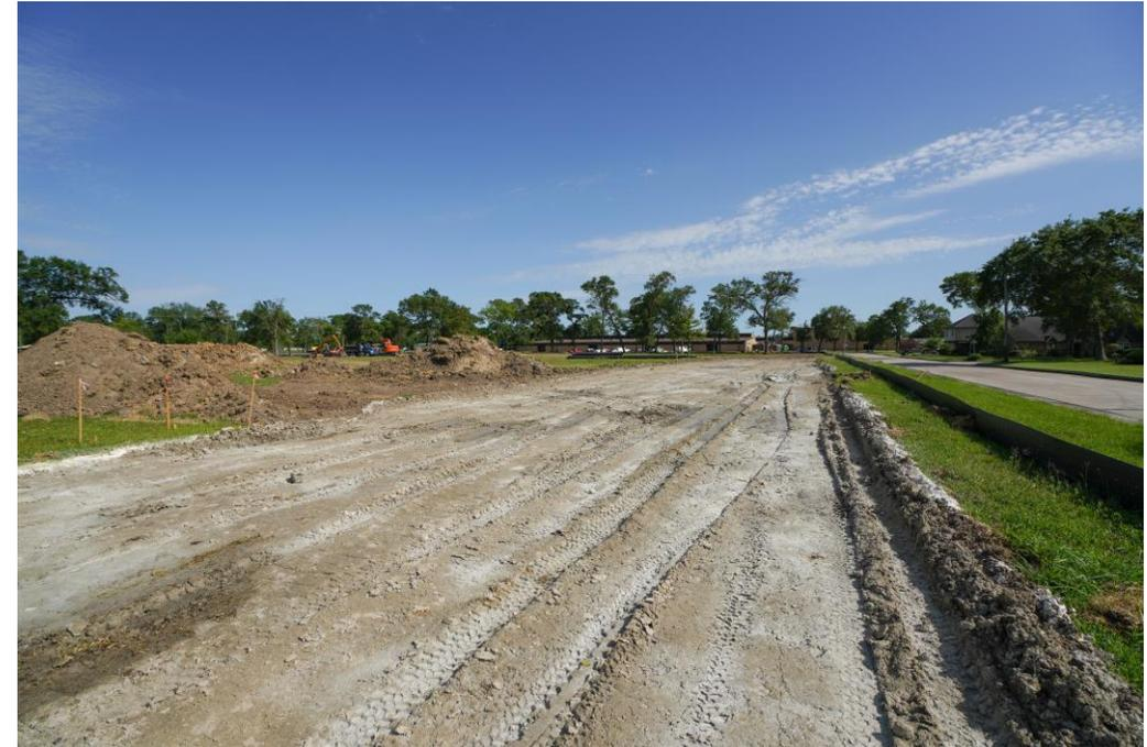
Lime stabilization is ongoing for the queueing lanes and new parking
