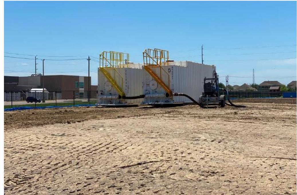
Frack tanks onsite to mix soil-stabilization material
