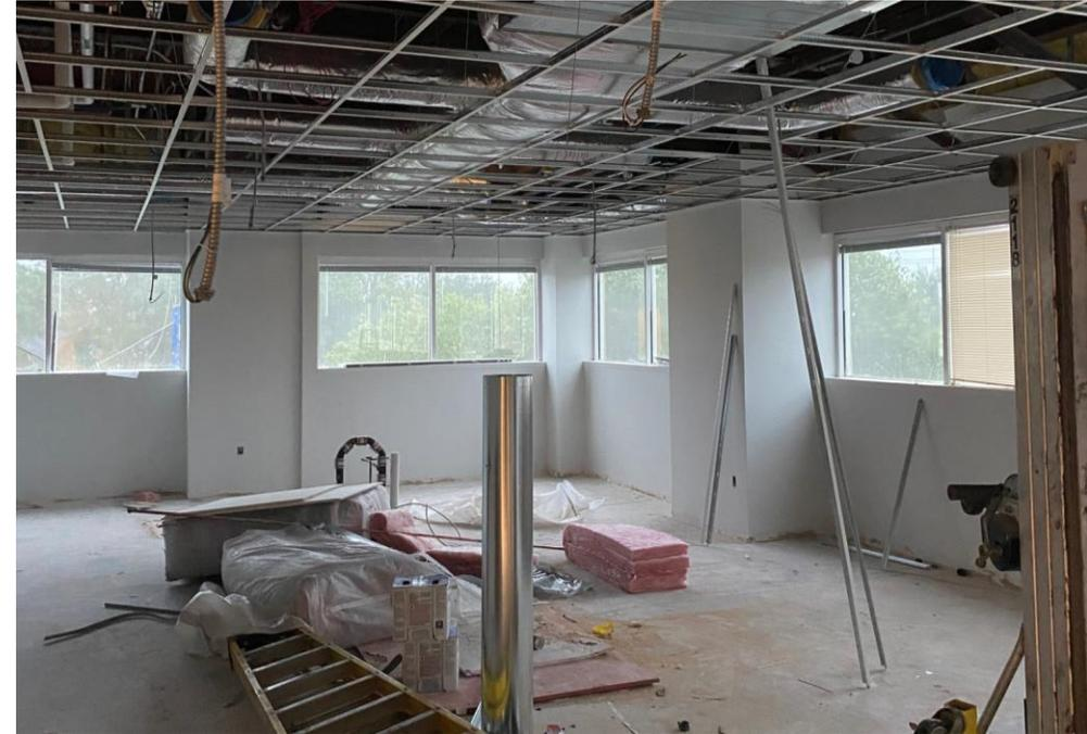
Metal framing & gypsum install is complete at the second floor, ceiling grid installation is underway
