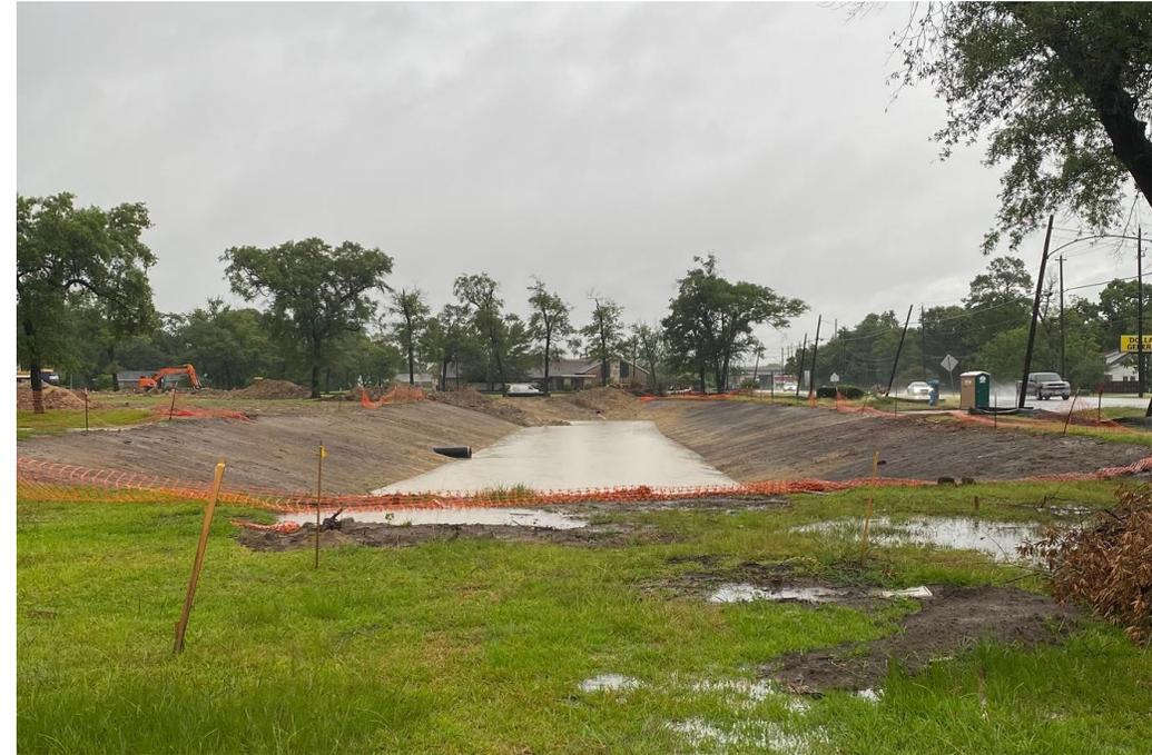
Excavation of new detention pond is complete
