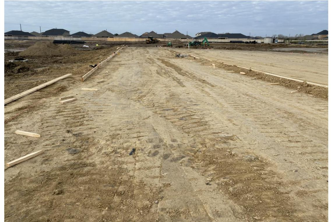
Final grading underway in preparation of concrete pour at parking lot
