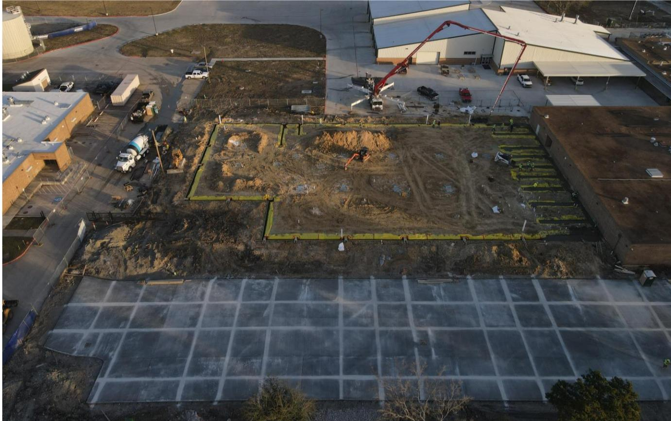
Aerial View – new concrete driveway poured; perimeter grade beams complete
