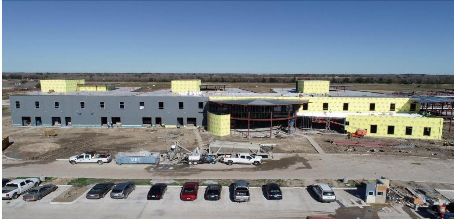
Installation of sheathing and waterproofing progresses
