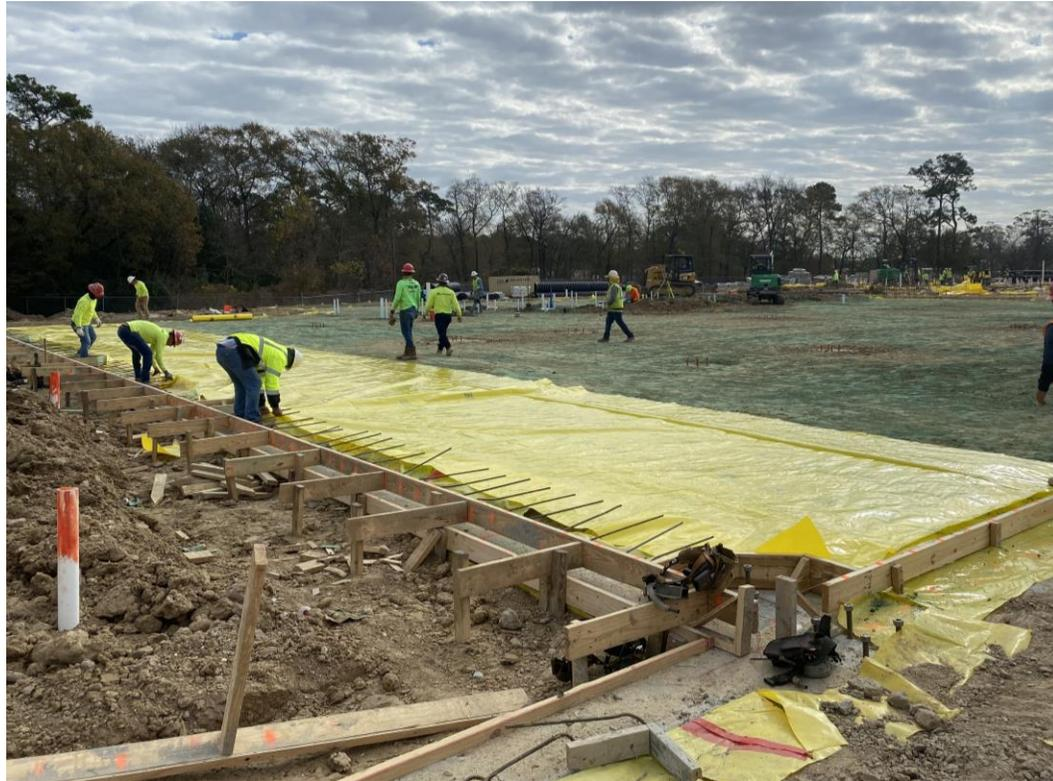
Moisture barrier installed in preparation of concrete pour at Area D of building pad
