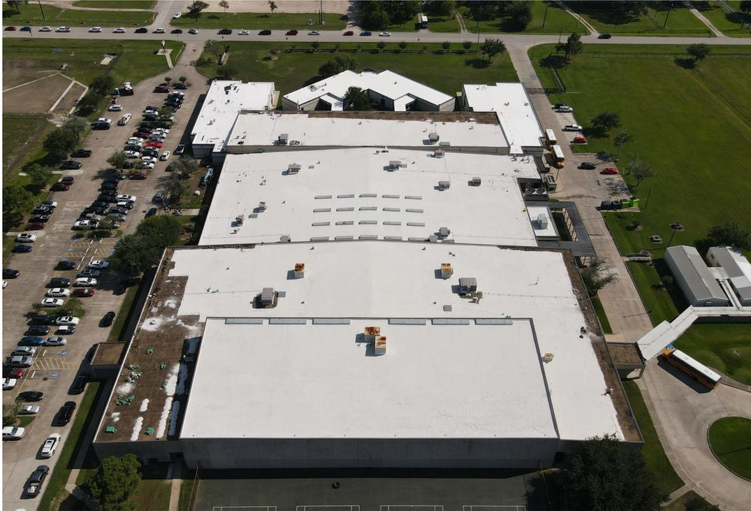
Installation of cap sheet almost complete at Gentry JS
