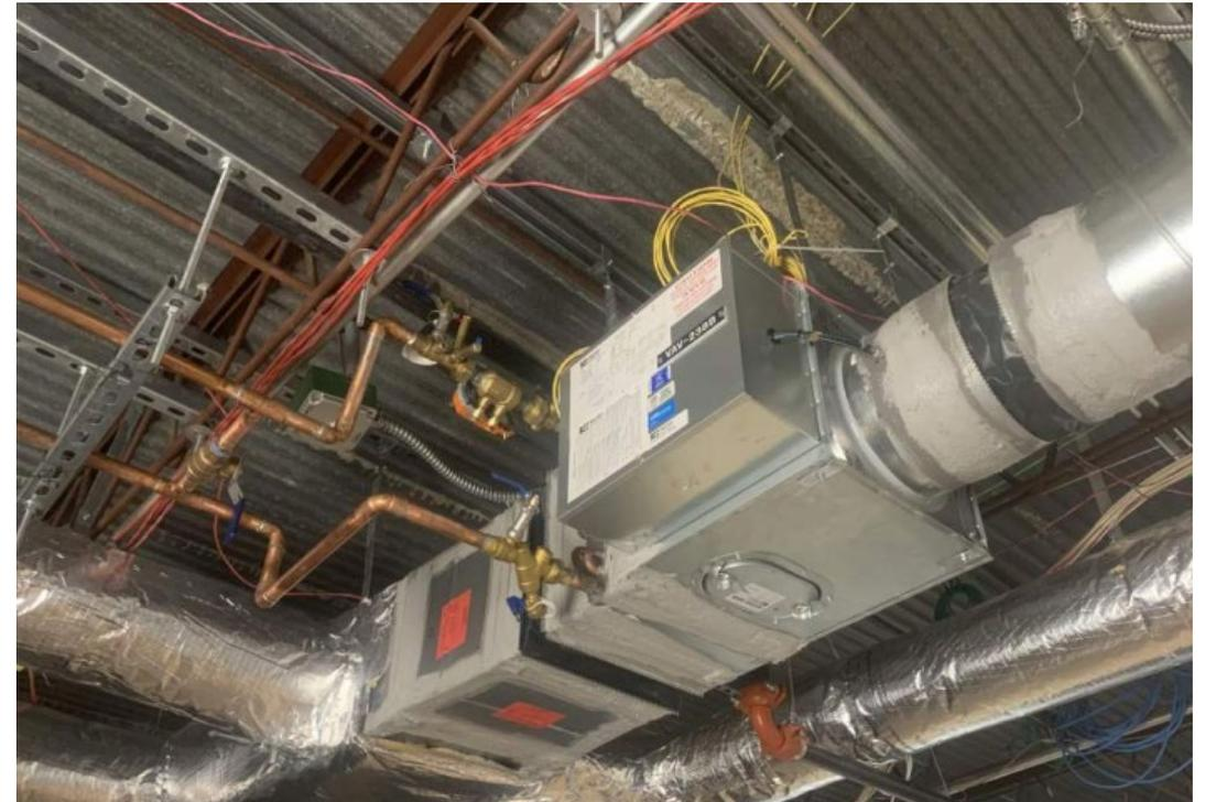
Ductwork tied into VAV boxes
