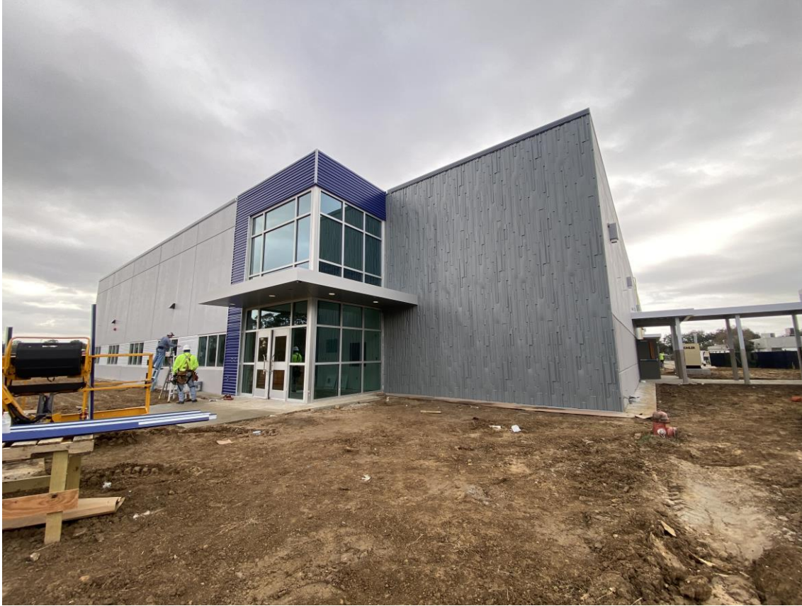
Metal panels and canopy installed
