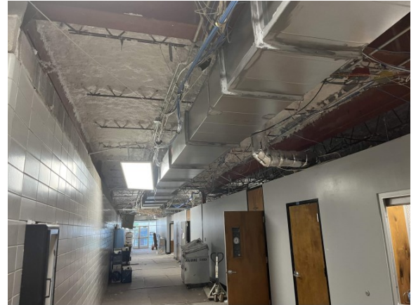
New Ductwork in Corridor
