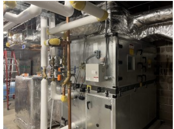
Insulation of Hydronic Piping
