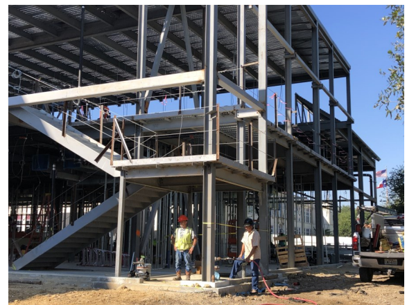
Structural steel stairwell at Lee HS
