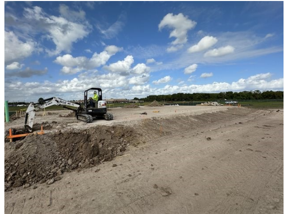
Building pad prepared for grade beams
