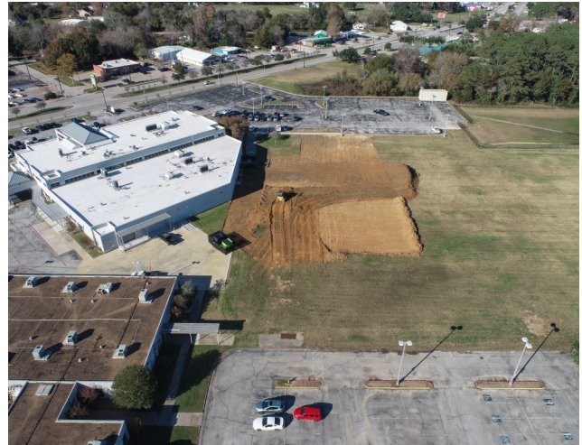
Project site rough grading underway
