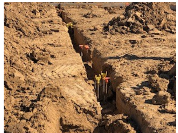
Grade beams & drilled piers underway
