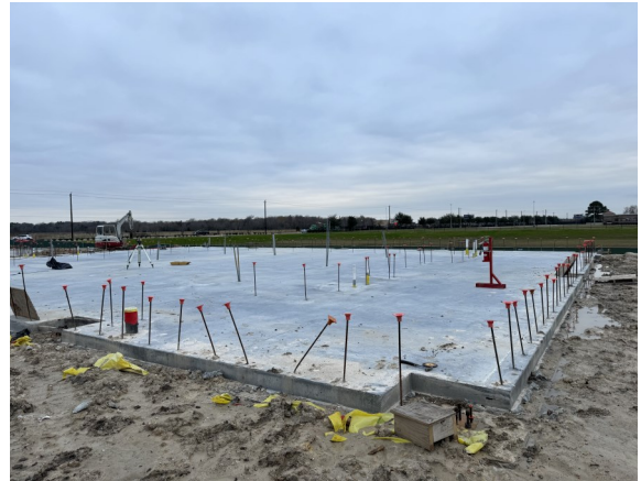
Building pad poured; awaiting steel
