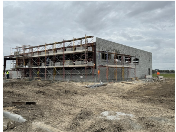
Exterior CMU installation underway
