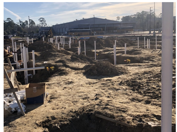
Electrical and Plumbing rough-in complete at building pad
