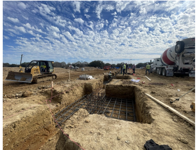
Re-bar installation for spread footings set in place
