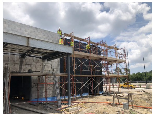
Waterproofing being applied over CMU
