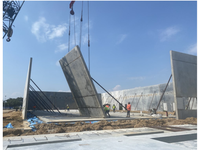
Erecting tilt wall panels
