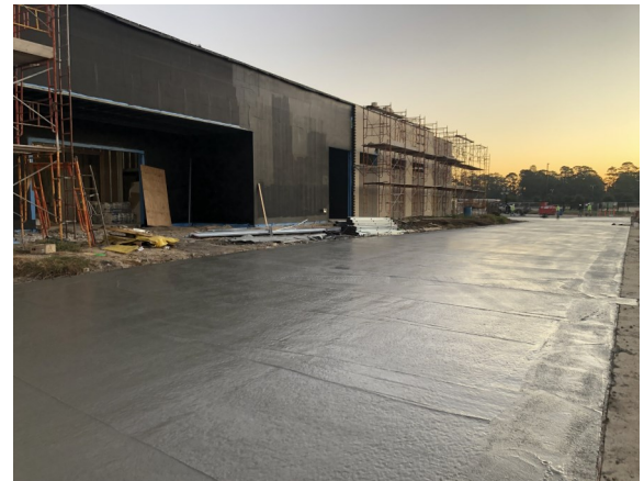
Concrete placement at front entrance
