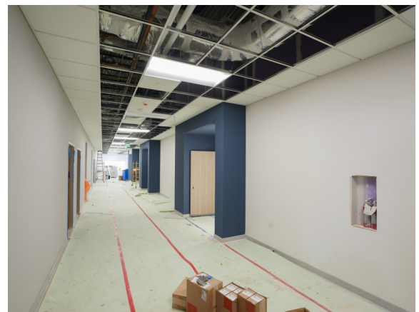
Vinyl Wall Covering Installed in the Corridor
