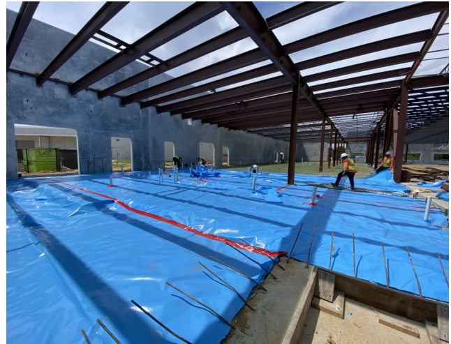
Vapor Barrier and Rebar Installation
