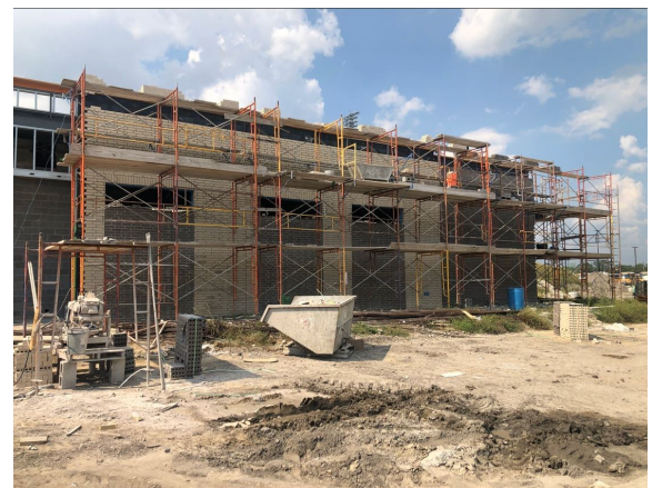
Exterior Brick Being Laid at South Façade
