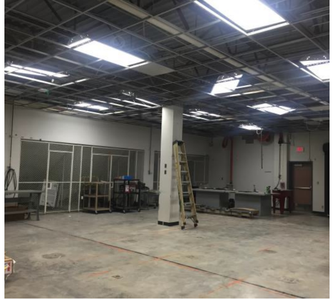
Demolition and cleanup at Horace Mann has taken place.
