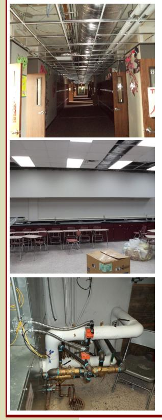
The new ductwork has been inspected and insulated. The grid has been replaced in the second floor hallways in the main building and east and west wings. Inspections are scheduled to facilitate the installation of ceiling tiles and lights. The first floor is scheduled to follow.
