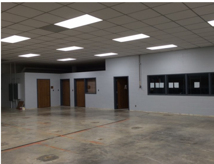
Demolition, renovations, new ceiling and painting is complete at Horace Mann Junior STEM Lab. The new flooring is in process at this time.
