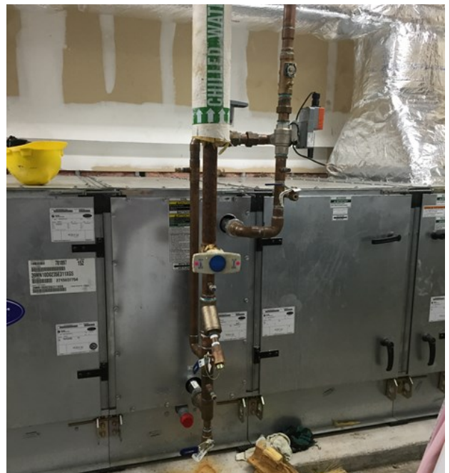
All of the new AHU's at Ashbel Smith have been piped and insulated. AC expected to start up by Friday, July 31st.
