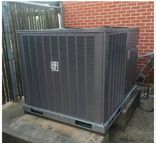
The DX unit at Cedar Bayou Special Education Building has been set.
