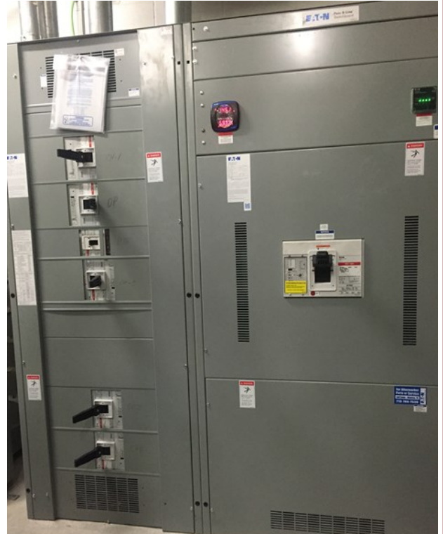
The new MSB at Horace Mann has been installed.
