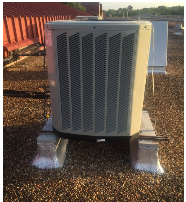
The new library DX roof systems have been installed at DeZavala, Harlem and Highlands .
