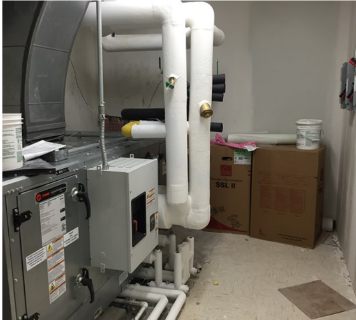
The new AHU piping and ducting has been connected at Hopper .
