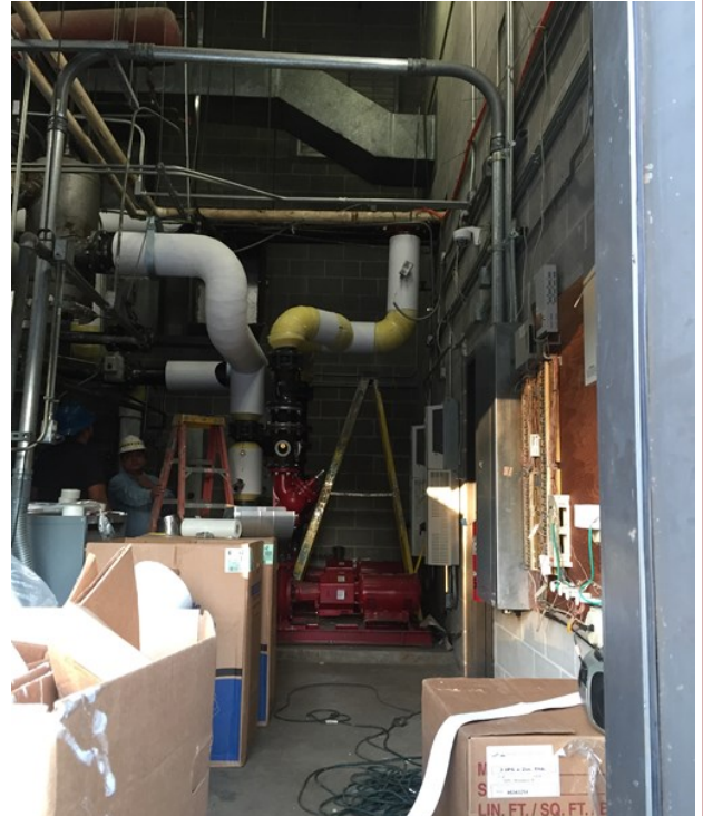
The condenser water piping is being installed at San Jacinto .
