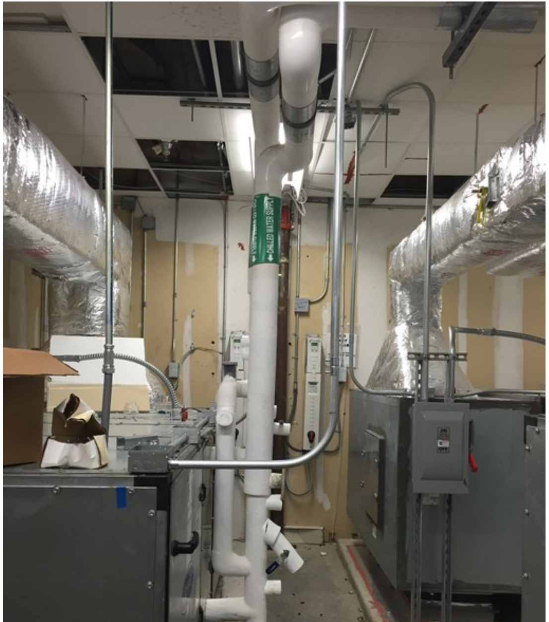
The new air handlers at Ashbel Smith have been installed.
