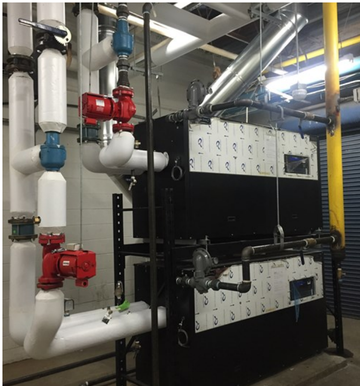
At Harlem the boiler piping has been insulated and flues have been installed.
