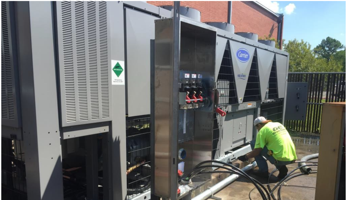
The new air chiller has been set at Cedar Bayou Junior School.
