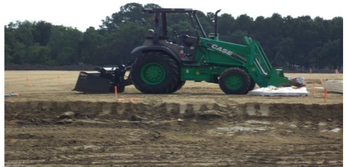
Building pad at N. Main and Archer Rd.
