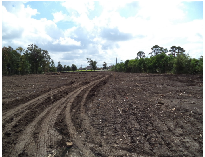
Clearing of the 146 site
