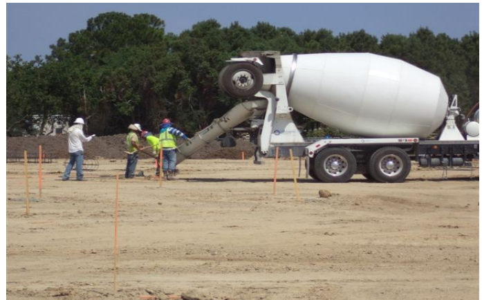
Building pad at N. Main and Archer Rd.
