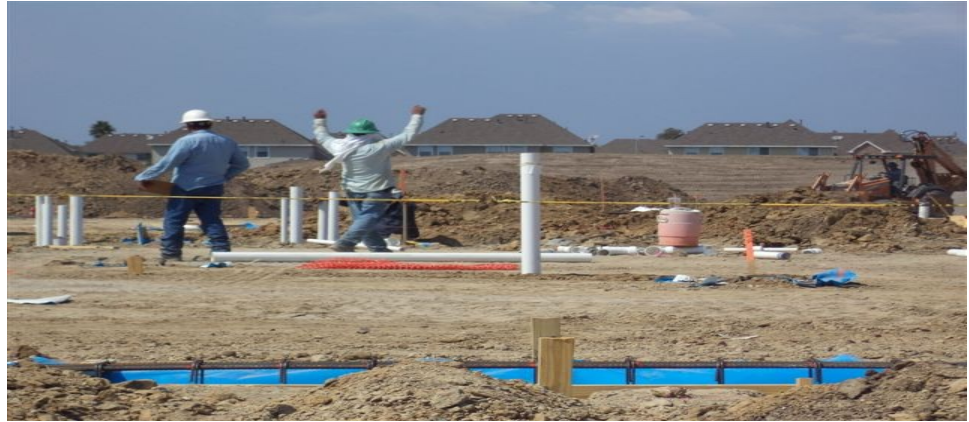
The New Elementary on Eastpoint is well under way.
