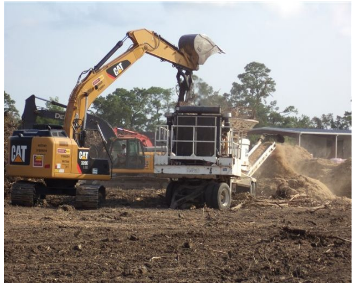
Clearing of the 146 site
