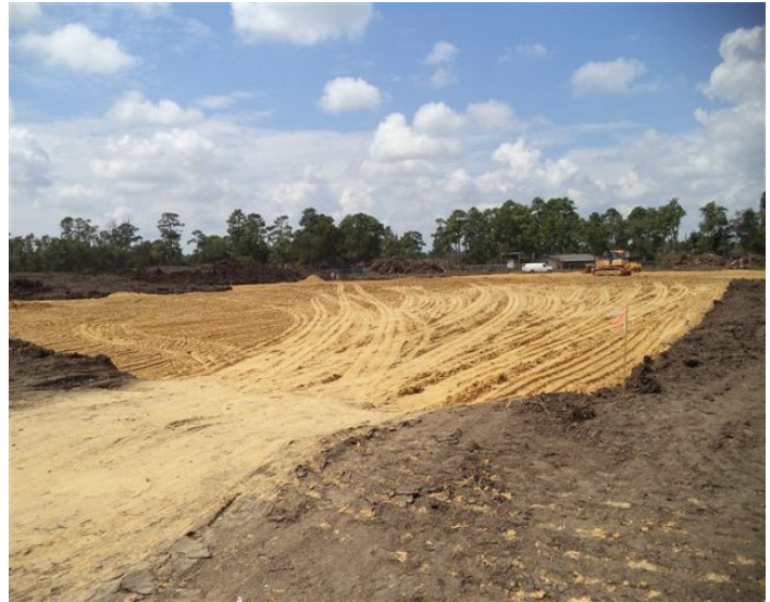
Preparing the pad at the 146 site
