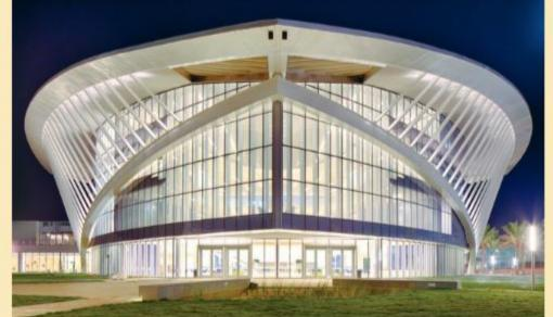
ing was limited, the structure "required extensive coordination for lateral brace frame layouts, gravity framing, and foundation design," explained the Thornton Tomasetti site. The building's iconic roof features a double-curved, steel-framed surface supported by a central spine girder and a series of wing beams. The spine girder is composed of two laced, wide-flange
